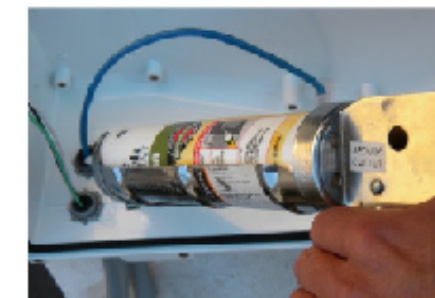
6) To assure an airtight seal, caulk around wires and cables, coating entire plug surface with sealant.
