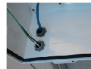
1) Pull wires to final installed length.
