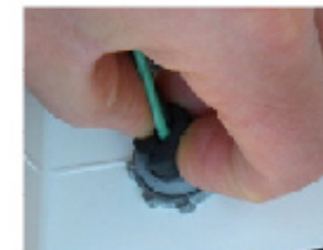
3) Pinch Plug to compress over wire, and insert into conduit feed mouth.
