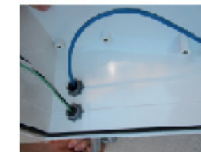
4) Push plug into conduit mouth with finger tips till it flush with outside of fitting.
